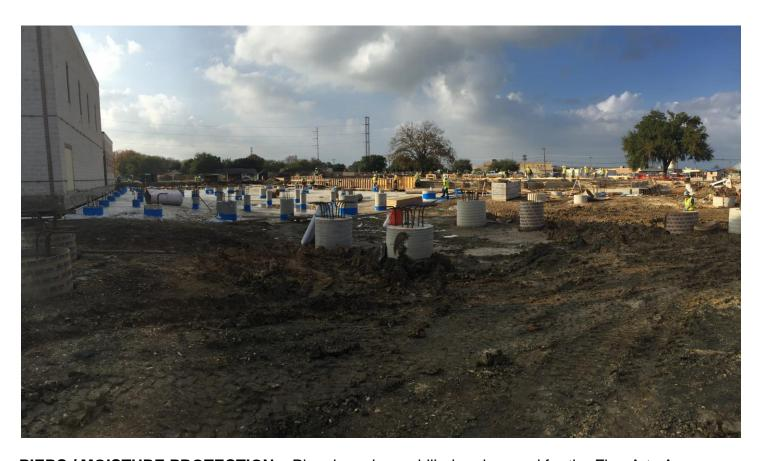
**PIERS / MOISTURE PROTECTION** – Piers have been drilled and poured for the Fine Arts Area between the new Auditorium and the existing Band Hall.
