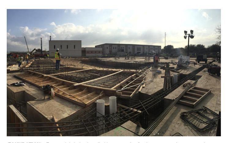
**FOUNDATION** – Formwork is being installed in preparation for the concrete placement at the Auditorium. Concrete was poured the following day on Wednesday December 16, 2015.
