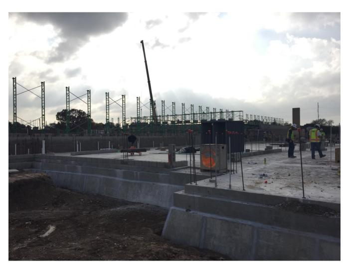
**FOUNDAION / UNDERFLOOR** – Concrete retainers are being placed and sealed to keep the soil and water from entering the under-floor area. Concrete walls being erected beyond.
