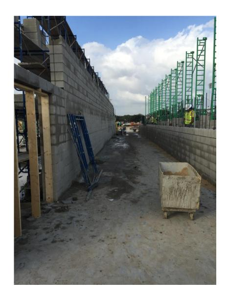
**WALLS** – Concrete block walls are being erected at the Gymnasiums.
